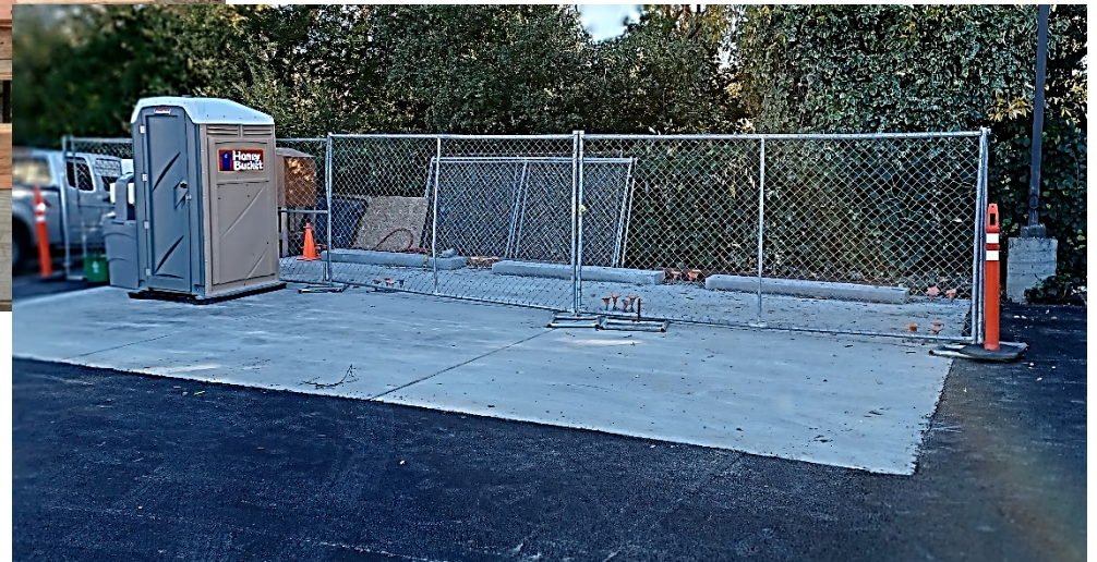
Trash Enclosure Slab and Apron
