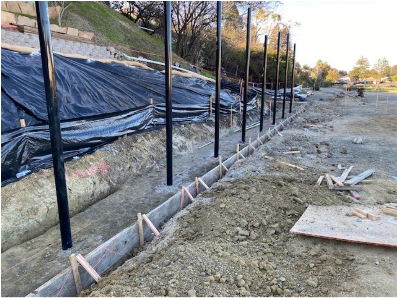
Basketball and Tennis Courts: Fence Post Installation, Retaining Wall Footing Prep Work
