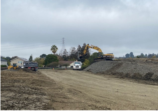
Excavator loading dump truck for spoils off haul
