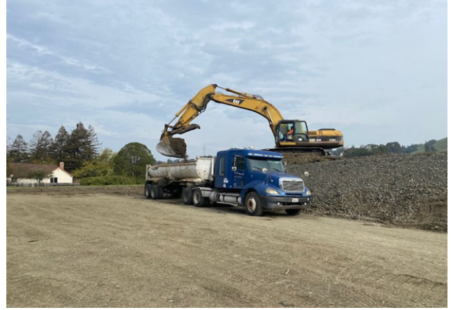
Excavator loading end dump truck for spoils off haul
