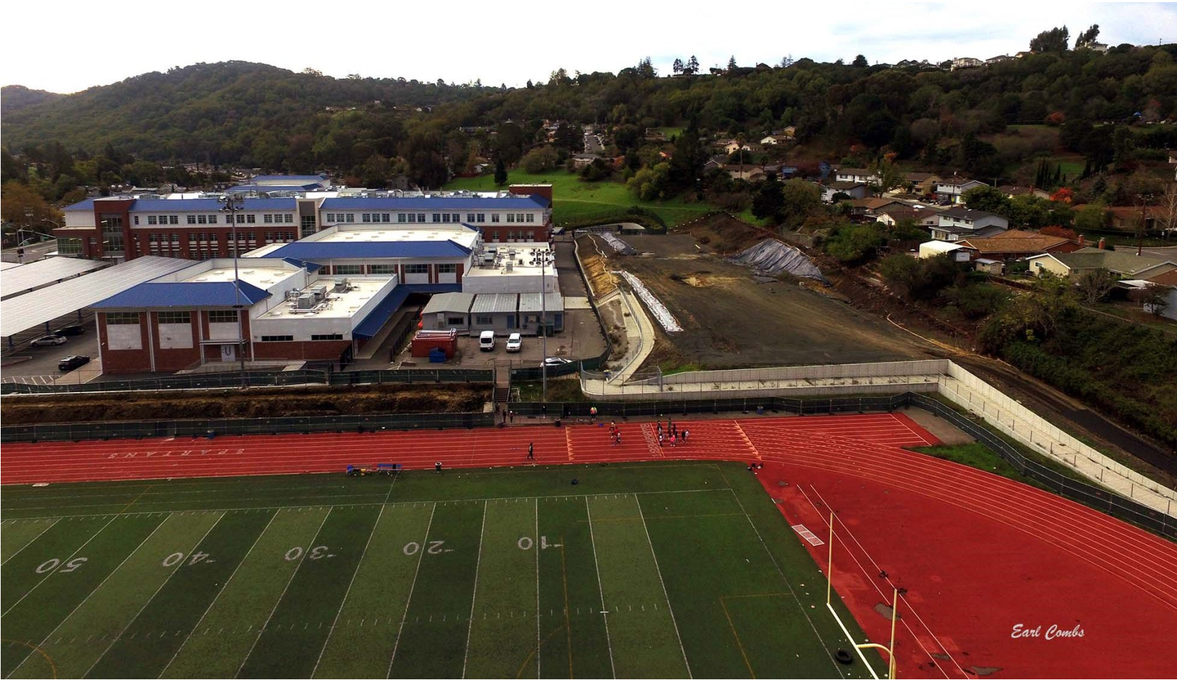
Basketball and Tennis Courts
