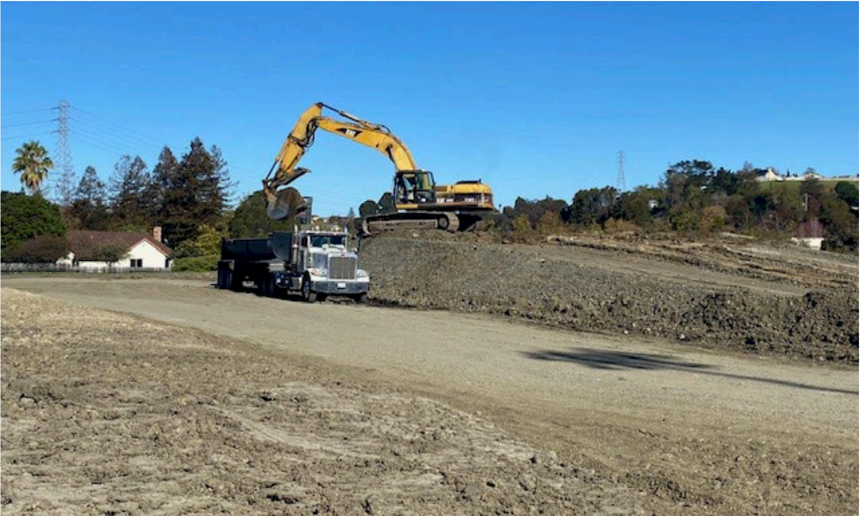
Baseball/Softball Fields: Removal of base material to establish subgrade
