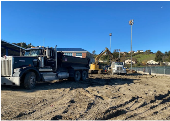
Excavator loading dump truck for spoils off haul
