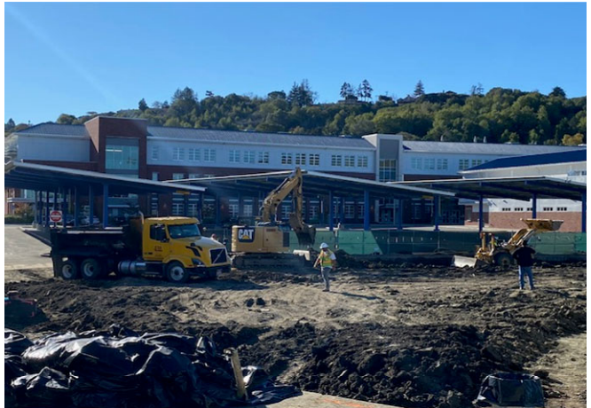
Excavator loading end dump truck for spoils off haul
